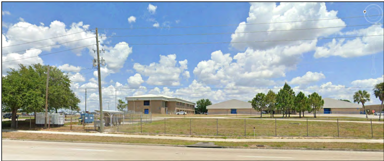
Figure 8: Existing Conditions of Sebring High School
