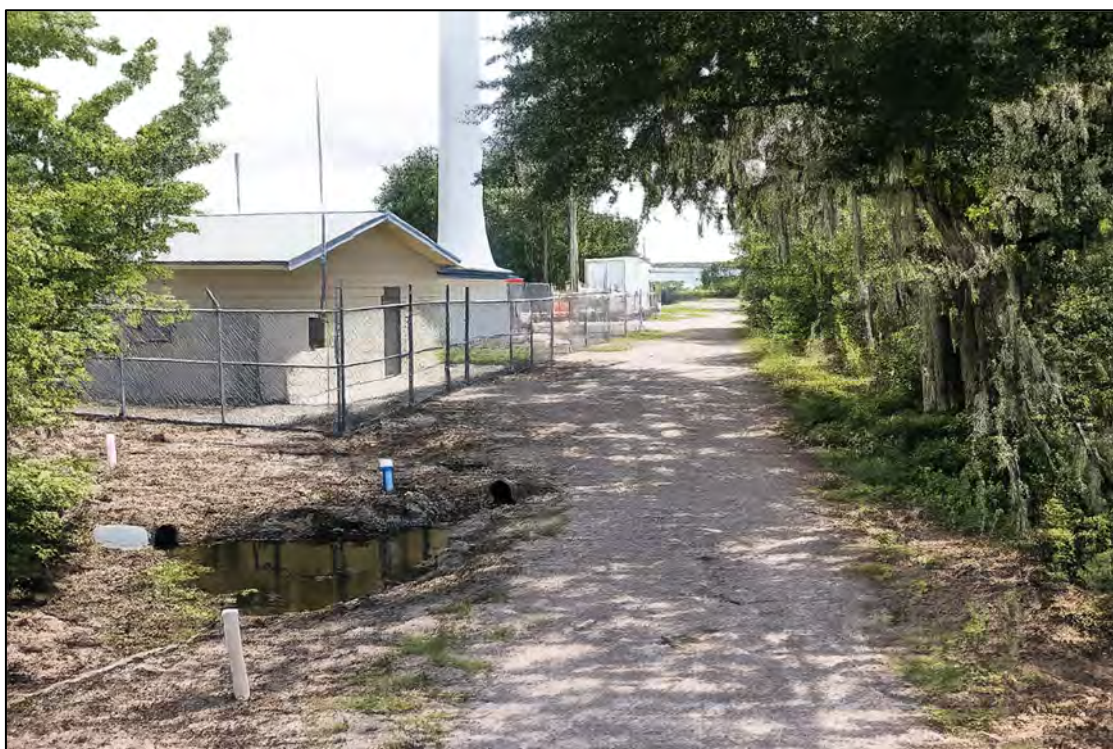
Figure 9: Existing Conditions of City of Sebring Fire Station #15c
