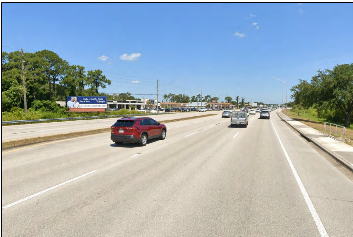
Figure 12: Existing Conditions of Highway 27 S
