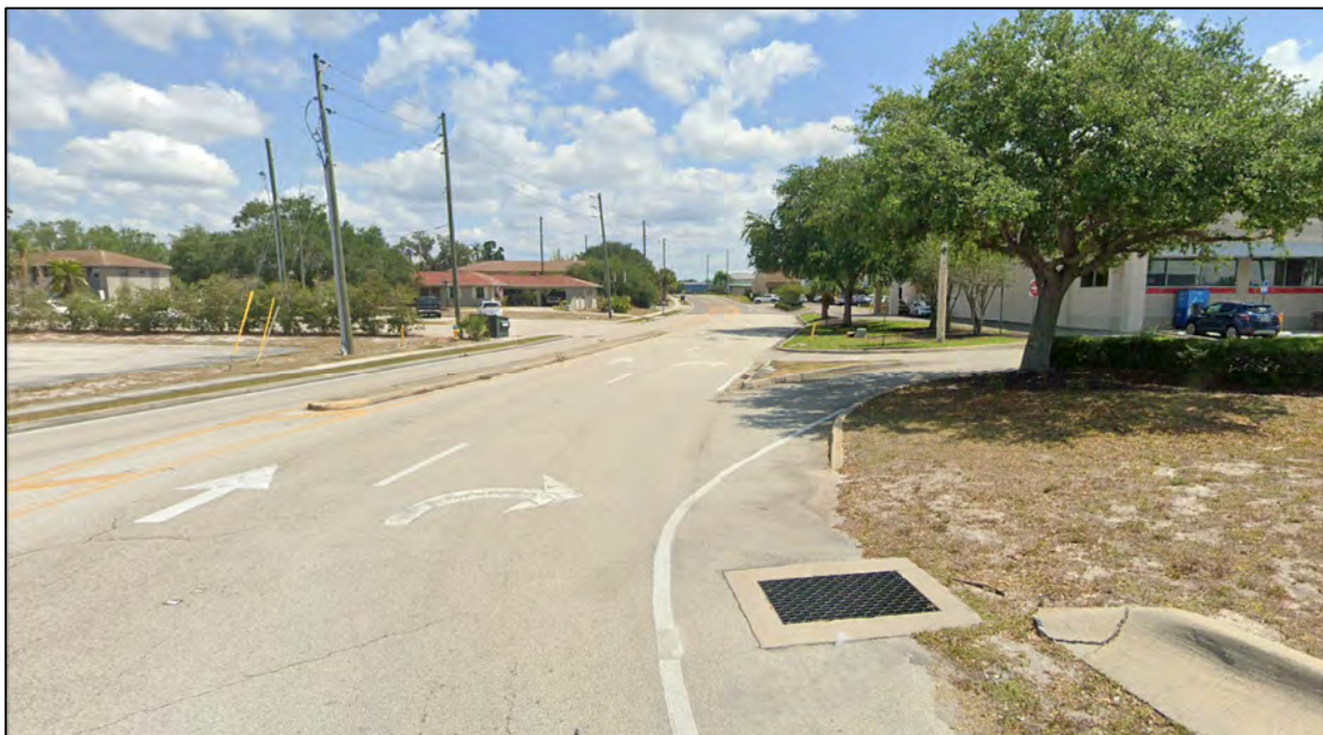
Figure 16: Existing Conditions of SE Lakeview Drive
