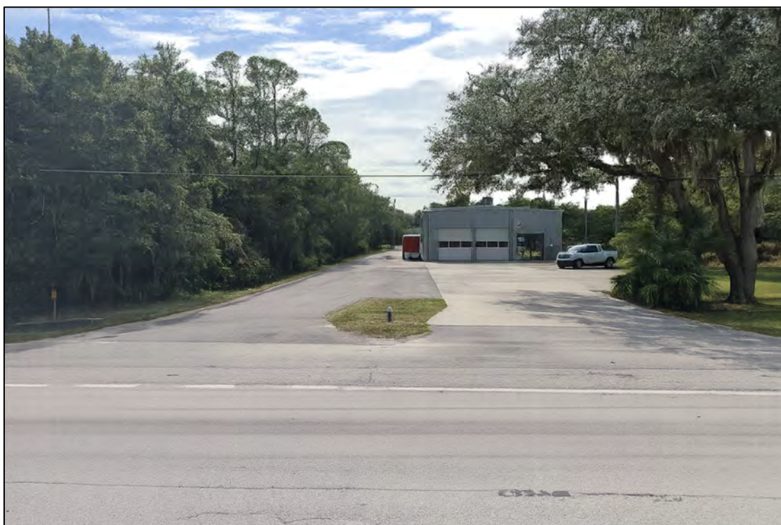
Figure 8: Existing Conditions of City of Sebring Fire Station #15
