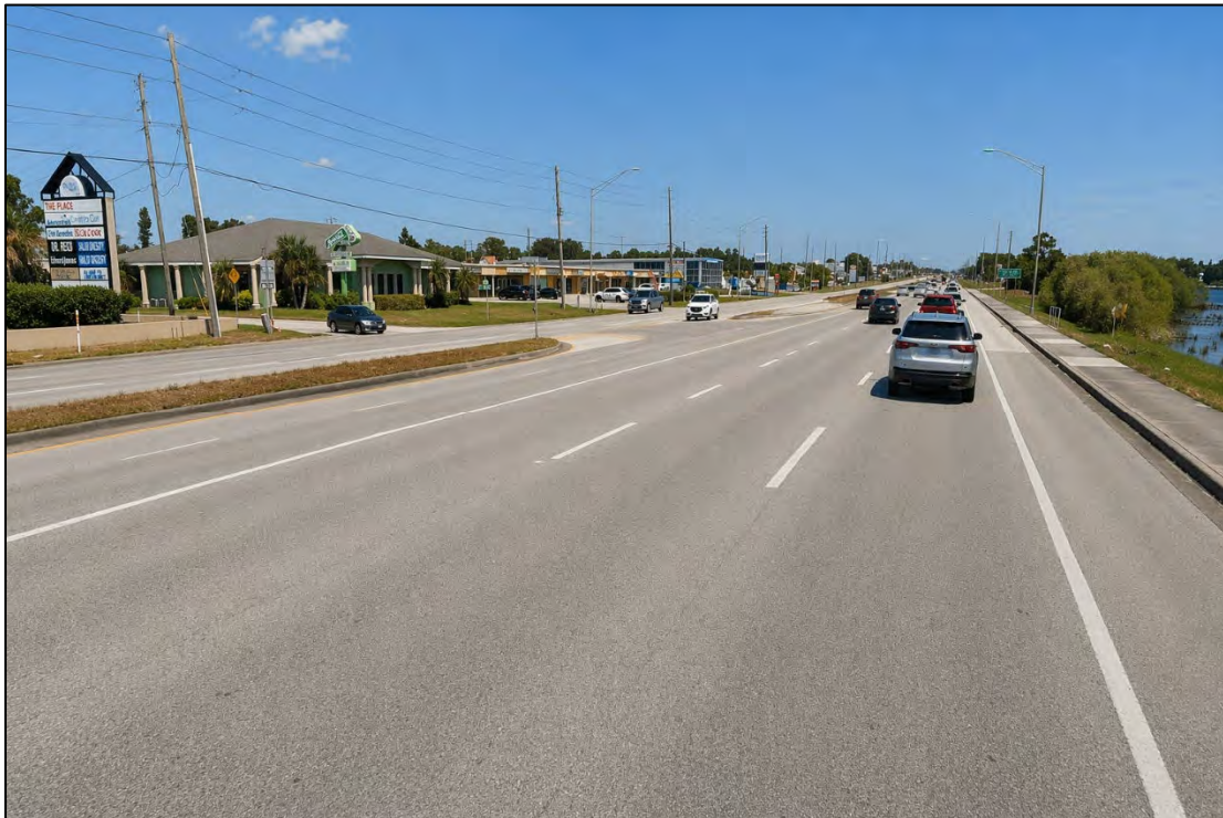
Figure 14: Existing Conditions of Ryant Boulevard
